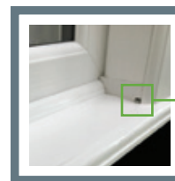
Drainage Channel
